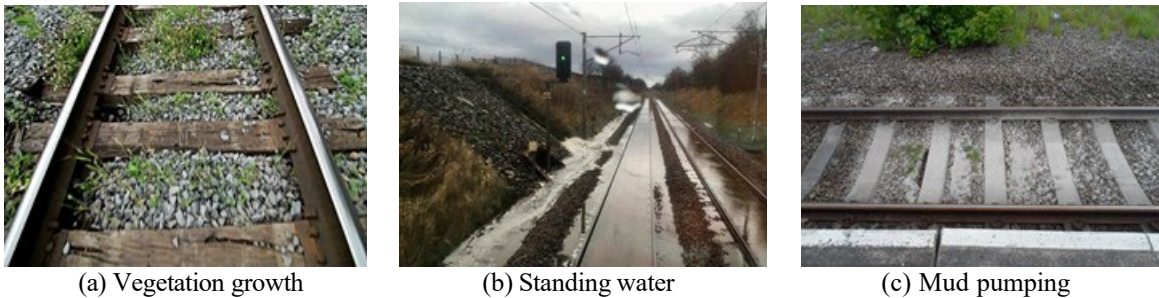
Figure 2.2: Rail Track Anomalies
