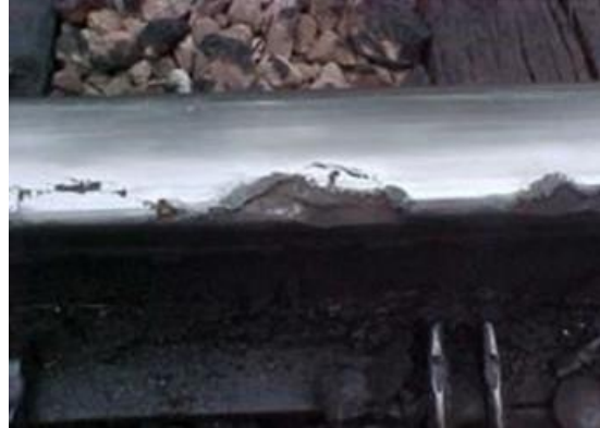
Side shells corrosion
