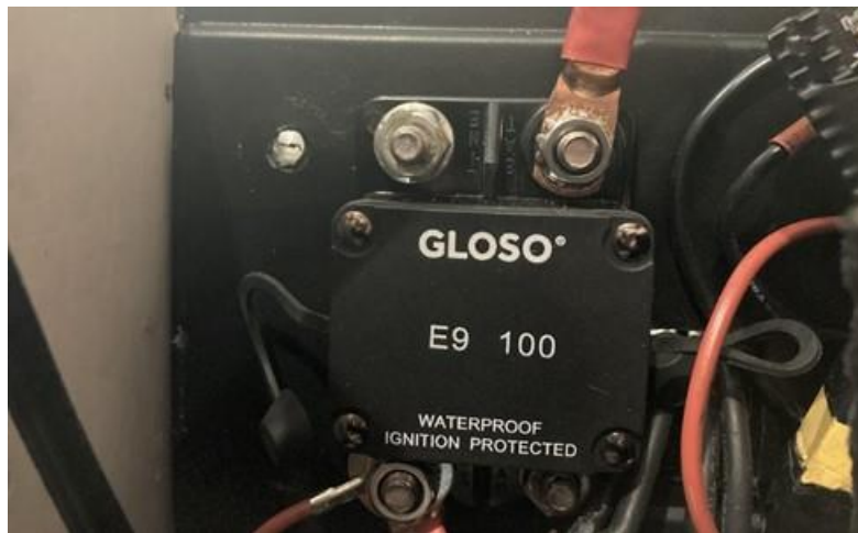
Figure 0-3: Installation of the auto-reset circuit breaker
