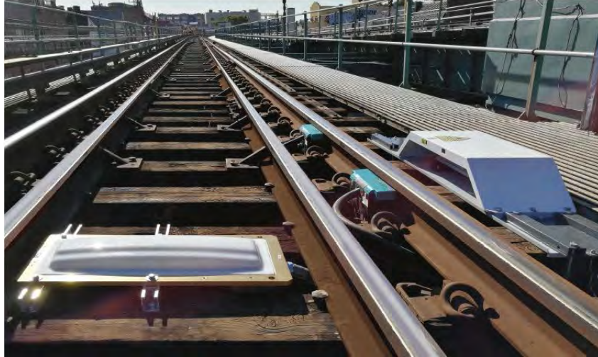
Figure 11 WID TBOGI site located north of 103 rd Street station (NYCTA).
