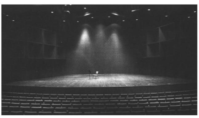
tower can be opened to permit stage lighting. The entrance doors on the downstage towers on each side are 5'-11" wide and the remaining towers have doors 5'-1" wide. All entrance doors are 7'-9" high but contain an obstruction in the form of a knee brace on each side of the opening at the top (see photo). The towers consist of a metal square-tube frame covered with particleboard and are painted "blackberry." They are 20'-0" high.
