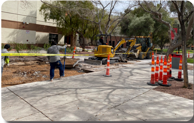
Picture on the Left: Sidewalk Removal by the Construction Crew
