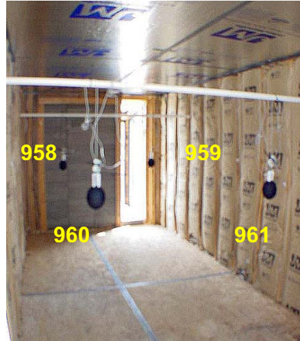
Fig. 2. Sunspace (SS) Interior View
