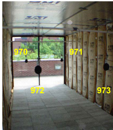
Fig. 5. Direct Gain (DG) Interior View
